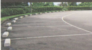
Large Parking area
